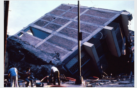
8-story frame structure with brick infill walls collapse due to resonance and duration of shaking - USGS
