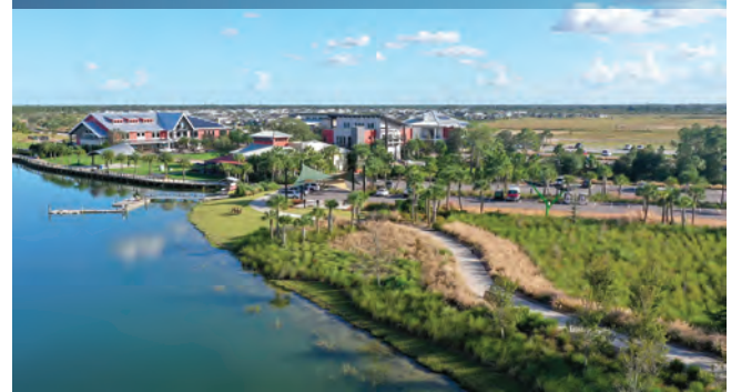
Not a single home in Babcock Ranch lost power or access to clean water when Hurricane Ian hit in 2022
