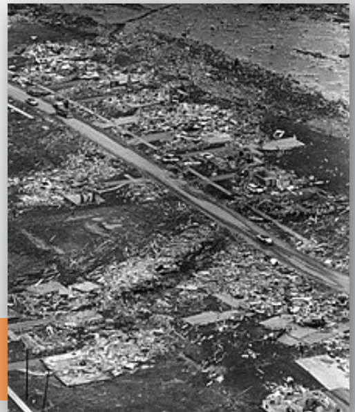
Damage in Toledo, Ohio, following the F4 tornado of April 11, 1965
