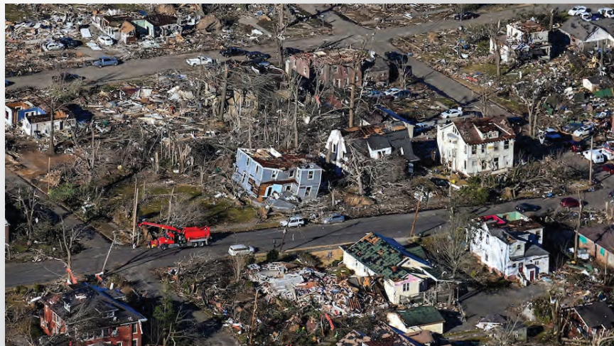
Homes destroyed by a tornado are seen from the air on Dec. 12 in Mayfield, Ky. (Joshua Lott/The Washington Post)
